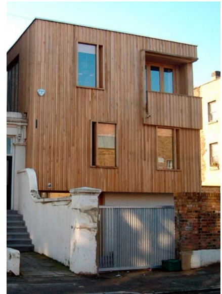
Lynch Architects Greenwood Road, Hackney, London
